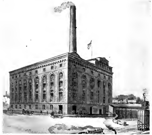
FIG. 2.—GENERAL VIEW OF CHRISTIAN STREET STATION, PHILADELPHIA.
